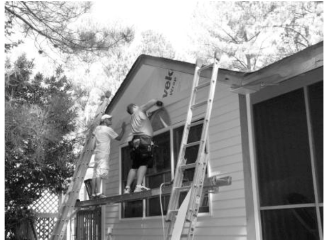
Work continues apace on new siding for the original cottages.
